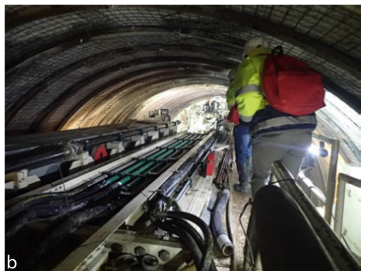
Fig. 12: The tunnel boring machine (TBM). a) The open gripper TBM. Approximately 70 % of the BBT is being built using mechanical excavation. b) The TBM will excavate 15 km of the exploratory tunnel in south direction.
