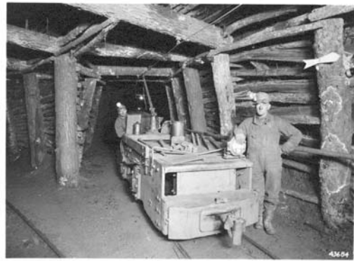
Fig. 9: Miners with a trolley locomotive in the Morris Lloyd iron mine, Marquette Range, Michigan, 1930s. Courtesy, Colorado School of Mines Library's Mining History Archive.
