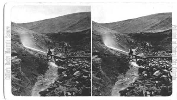
Fig. 2: A stereopair depicting hydraulic mining of gold placer deposits in Russell Gulch, Colorado, late 1800s. Collier's Rocky Mountain Scenery company produced stereopairs of Colorado scenery for sale. Courtesy: Colorado School of Mines Library's Mining History Archive.
